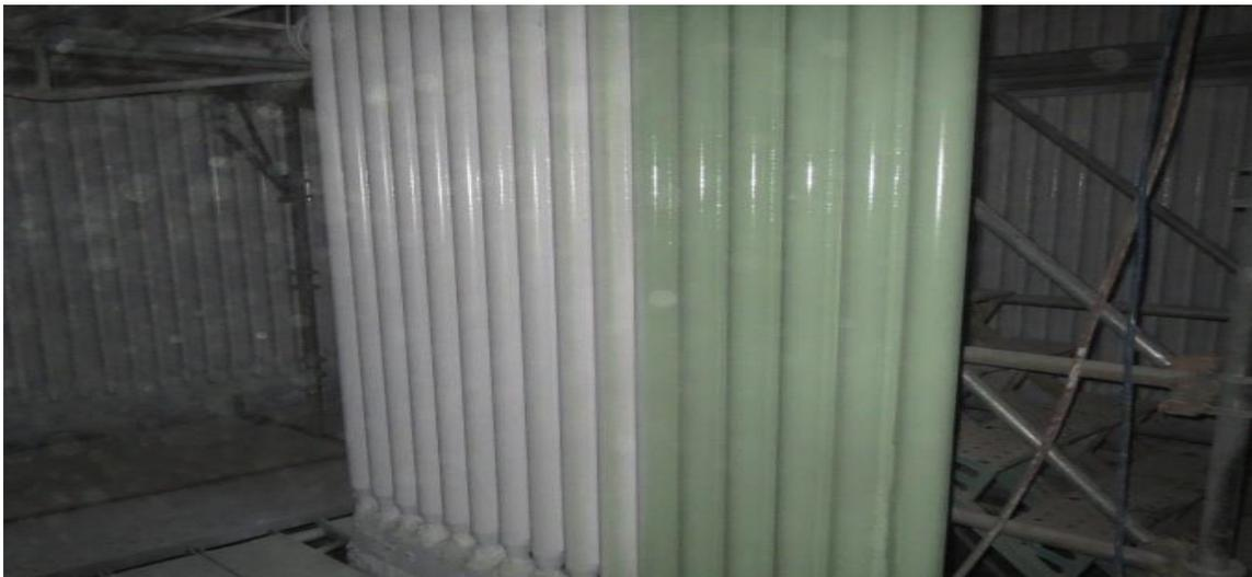
CFB (water wall) condition upon inspection after one year run in CFB boiler
